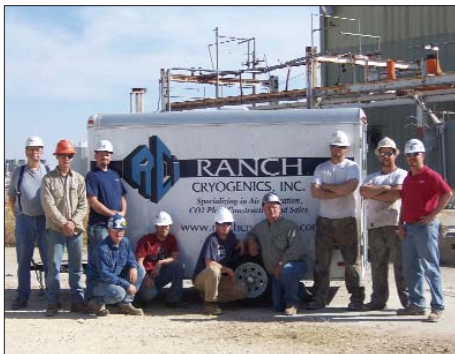
RCI recently completed the disassembly of a 120 TPD liquefier in West Texas
