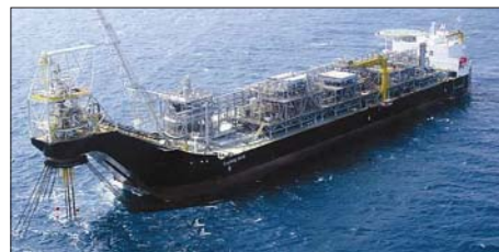
Velocys joins Toyo Engineering and MODEC in developing GTL facilities for off-shore applications.
